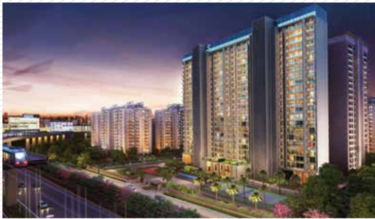
PLATINUM TOWERS, IFFCO CHOWK, GURGAON
